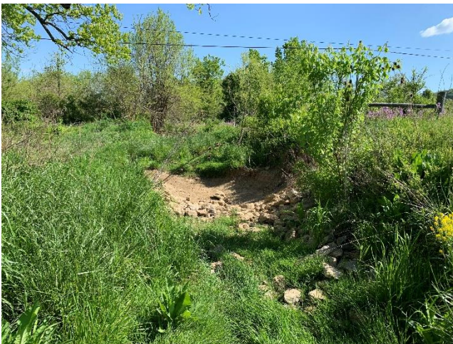
5/11/2021 – 5-year site inspection
