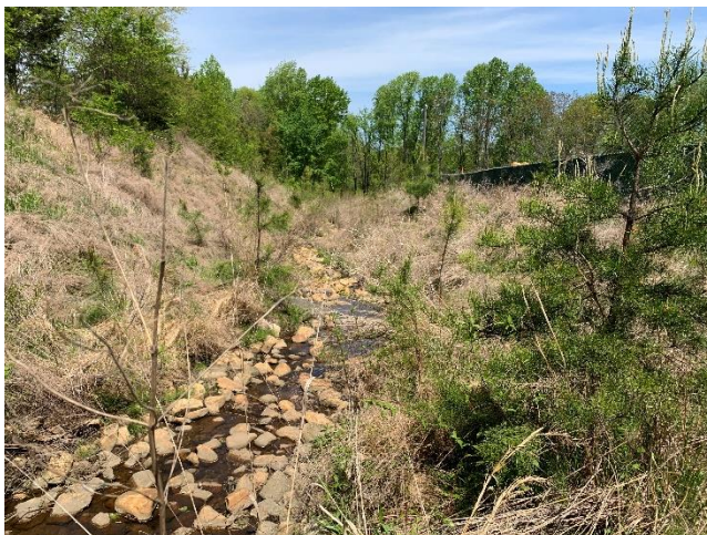
4/23/2021 – 5-year site inspection
