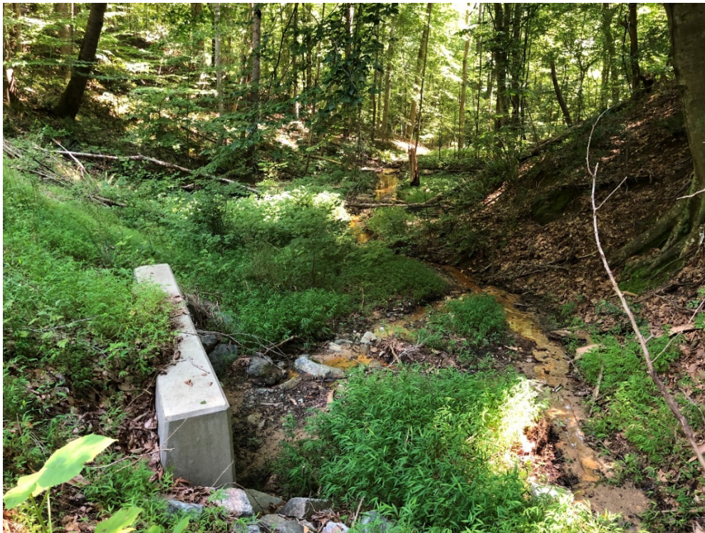
Photo 4: Outfall channel downstream of outlet pipe (2021)
