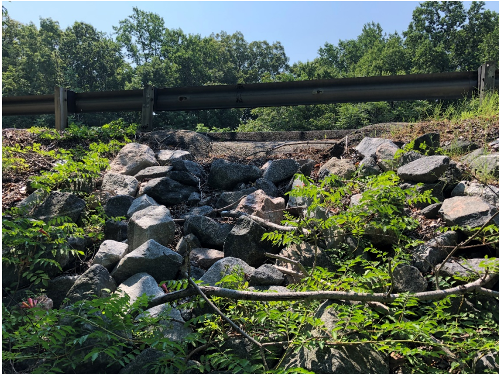
Figure 2: Outfall stabilization project during inspection (2021)
