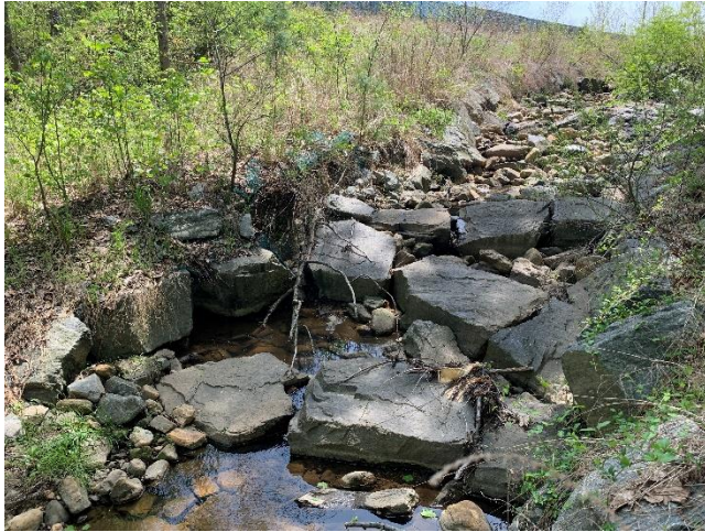
High flow flanking around the right side of S12.
