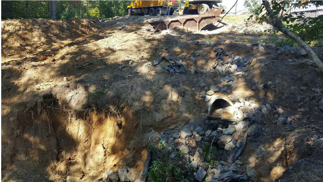
Figure 2: Banks of outfall channel before stabilization project was implemented (prior to 2021)
