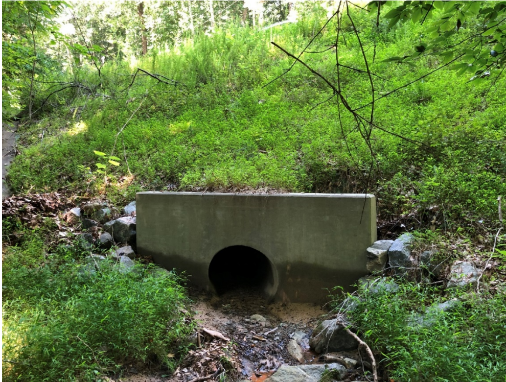
Photo 3: Downstream of Pipe Outlet (2021)
