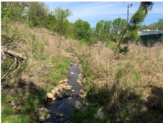
4/23/2021 – 5-year site inspection
