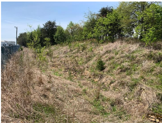
4/23/2021 – 5-year site inspection
