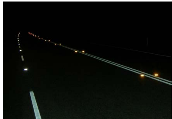
Figure 4.5.2.3 - Raised Pavement Markers
